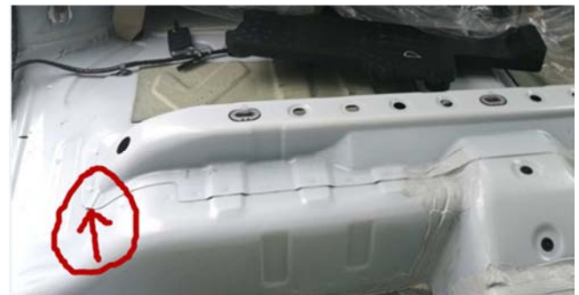
Figure 4. The water inlet at the right side of the middle floor.
