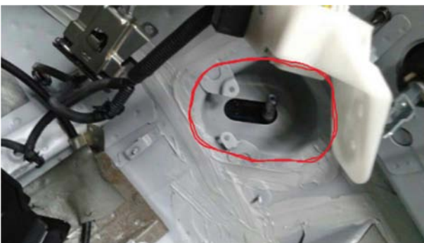
Figure 7. Water inlet at the through-hole position of the steering column.
