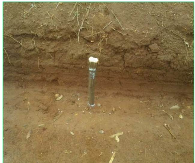
Figure 2. Peg placement at 0+500 on Kuywa-Kopsiro Road.
