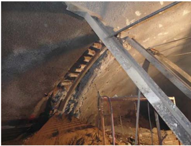
Figure 1. Tunnel hole to support.
