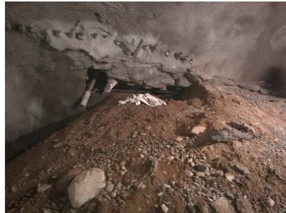
Figure 8. Cavity backfill grouting.
