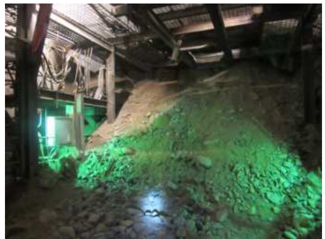
(b). Constraints collapsed
