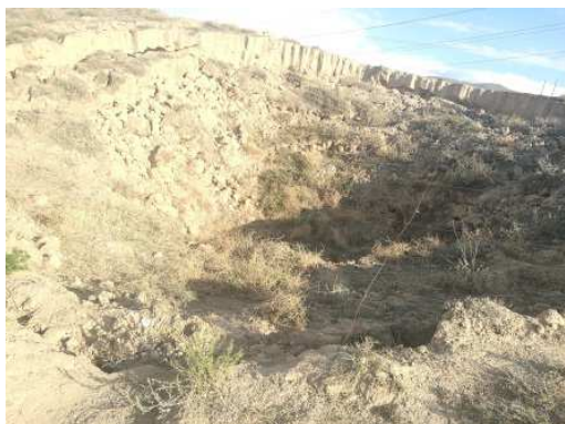
(f). The surface of the roof.
