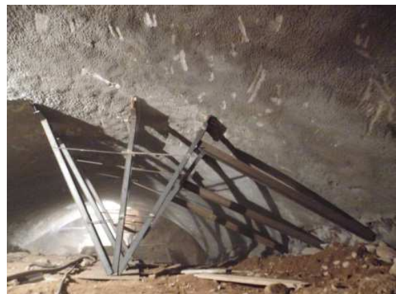
Figure 9. Temporary support in the hole.
