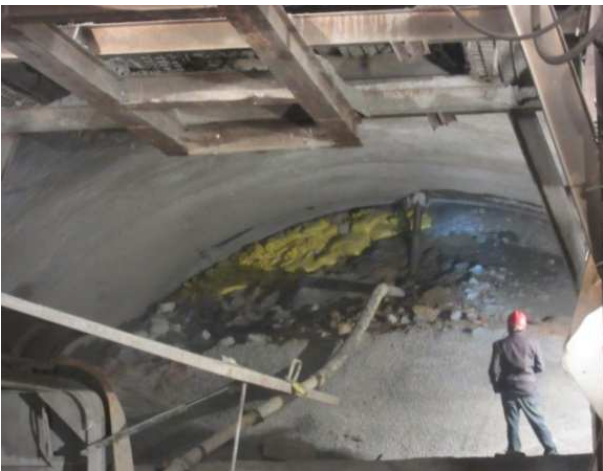
Figure 7. Sandbag plugging and backfill of the grouting.
