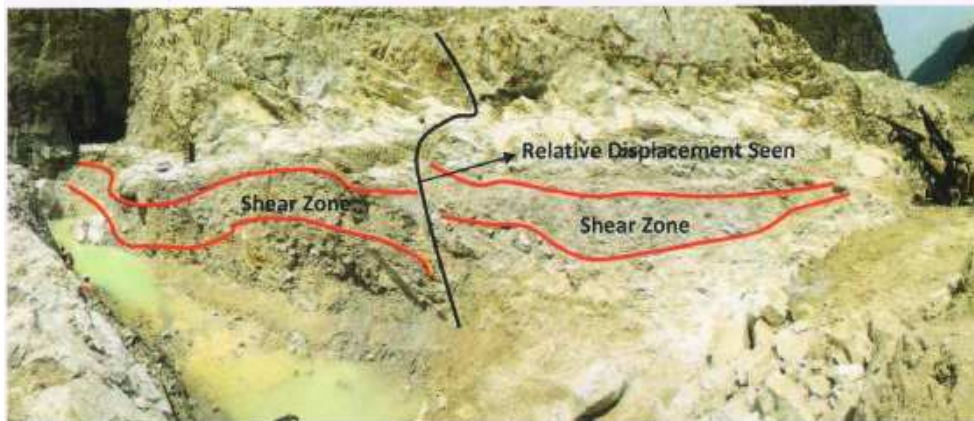
Figure 2. Shear Zone at Left Side of Excavated Trench.
