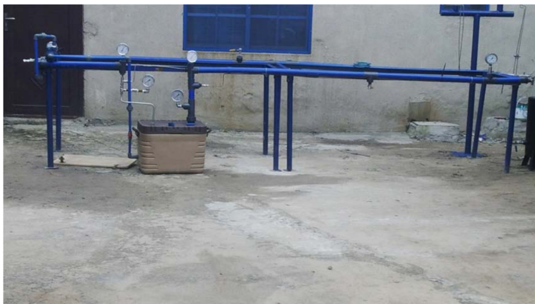
Figure 10. Frame Work of Laboratory Loop during construction.
