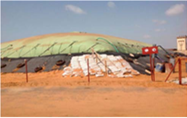
Figure 2. Photo SOGAS Dakar Tarpaulin Digester.
