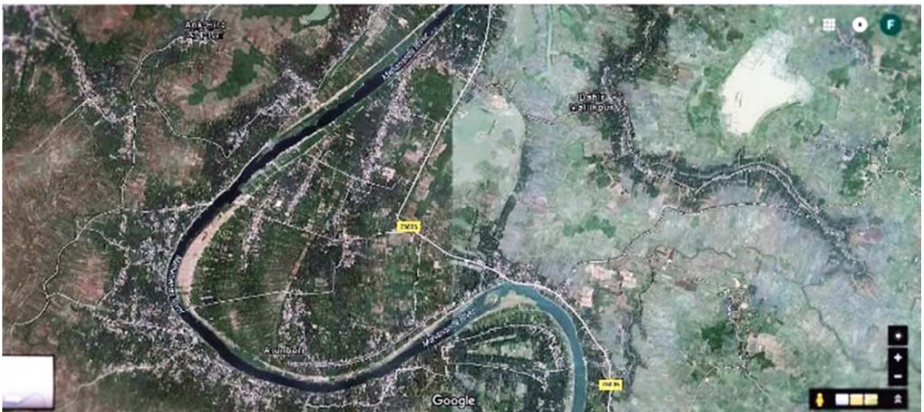
Figure 1. Location of Mahananda earthen embankment.
