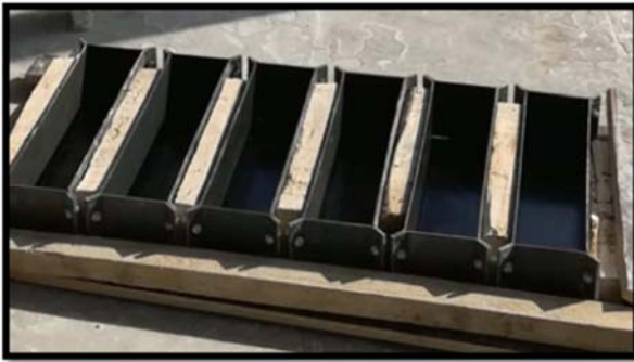
Figure 5. RCC Sample formworks.
