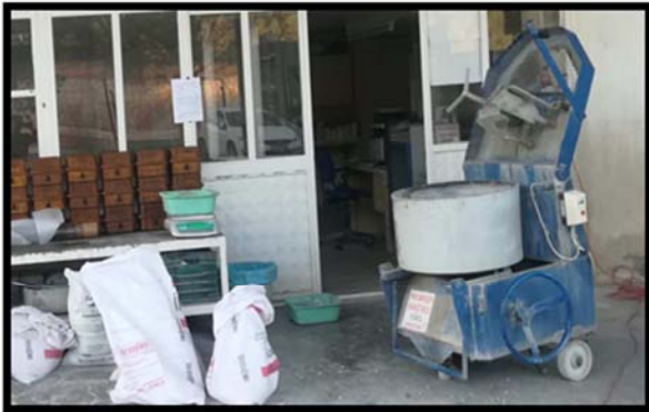
Figure 6. RCC Materials mixing.
