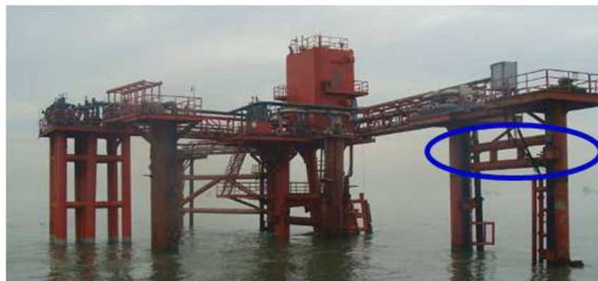
Figure 7. Tubular frame in offshore platforms.
