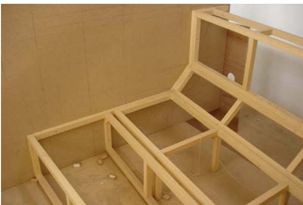
Figure 6. Wooden framing of a berth is placed with 40 cm. distances.
