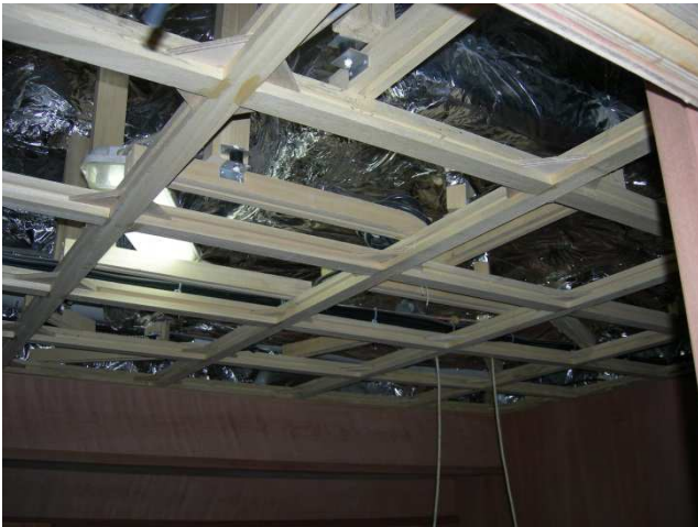
Figure 2. Ceiling structure is a grid system of wooden elements.
