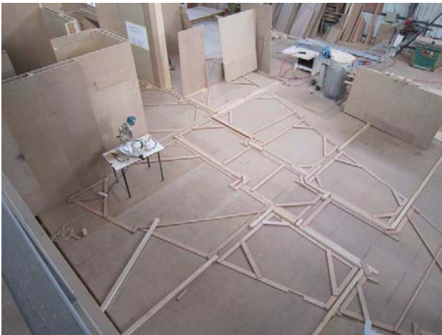
Figure 5. Plan layout of partition walls are made by wooden guides.
