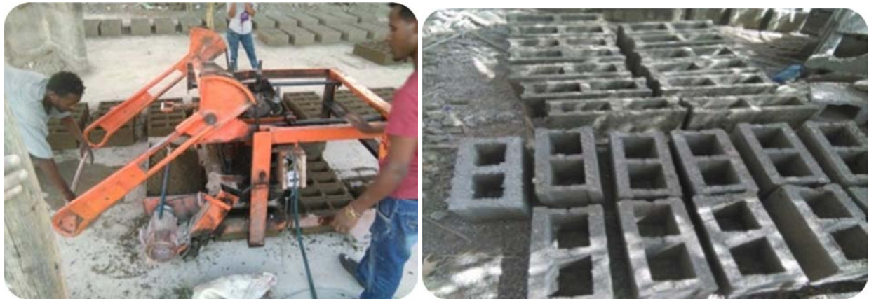
Figure 7. Production process of Papercrete hollow block.
