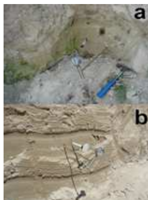
Figure 7. Measurement of soil moisture content in TBJ slope of G unit. a) monitoring point 1 in Fig. 9 (TMS1, left side of photo) and suction (tensiometer, right side of photo). b) photo is point 2 of Fig. 9 in Mejicanos.
