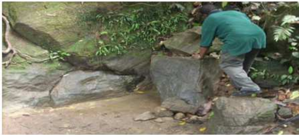
Fig.13. Water seepage from fractures in schist at Olum
