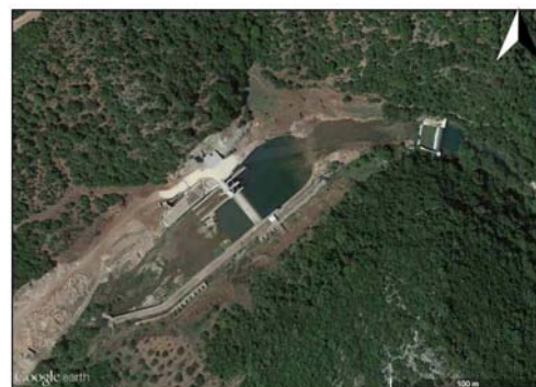
Figure 3. View of the constructed dam (Google Earth Pro/ Terra Metrics).
