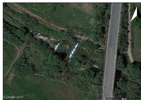
Figure 4. View of the transversal terraces after the dam (Google Earth Pro/ Terra Metrics).
