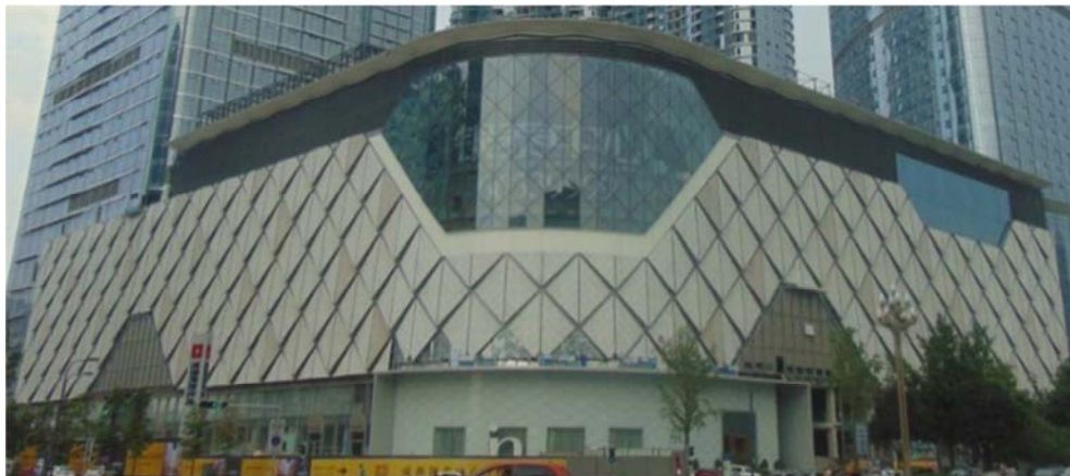
Figure 5. Overall effect of stone curtain wall of commercial annex building of Chengdu Yintai Center.
