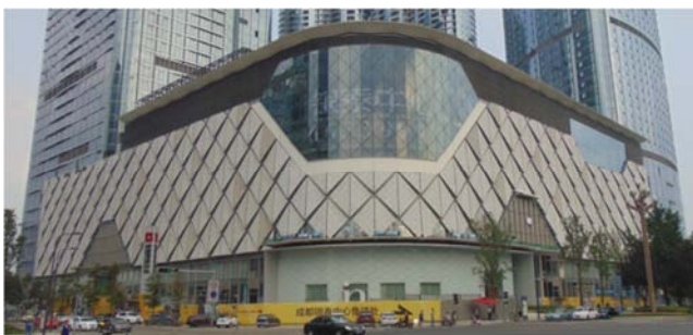
Figure 16. Picture of stone curtain wall of Chengdu Yintai Center.
