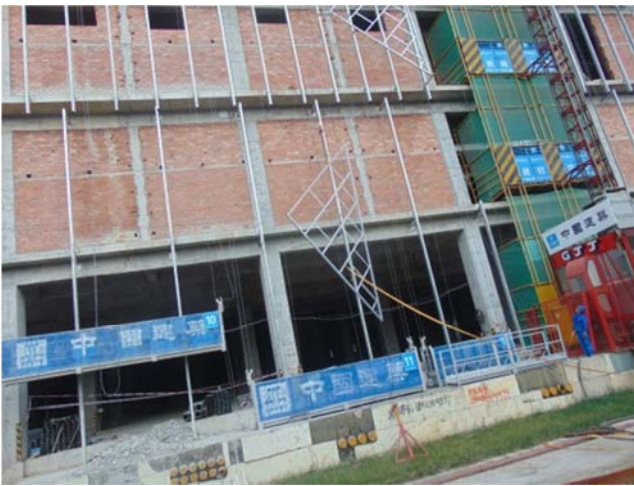
Figure 11. Overall lifting of triangle frame.
