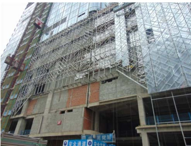
Figure 12. Picture of stone sub-keel triangle frame installation.
