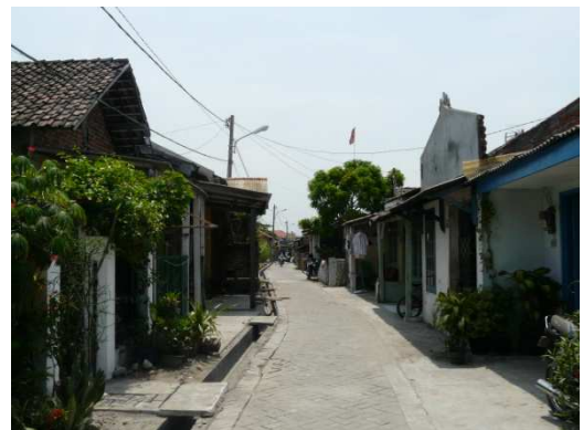
Figure 4. Open drain and pavement footpath in informal settlement
