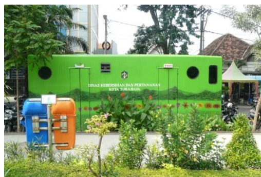
Figure 9. public toilets which cannot be used by disabled people.
