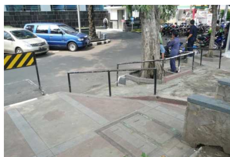
Figure 10. Ramps that cannot be used independently by wheelchair users.
