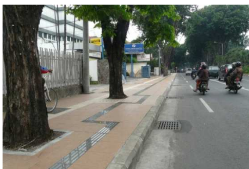
Figure 7. Tactile paving with wrong color, placement, and slippery material
