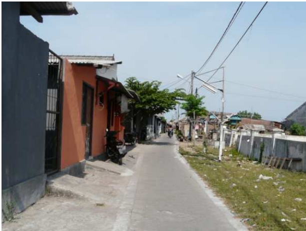
Figure 1. Unclear separation between footpath and roadways
