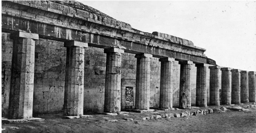
Figure 14. Is showing a group of free standing columns supporting the retaining Wall of the mountain at Deir el-Bahari." Reference: [19].
