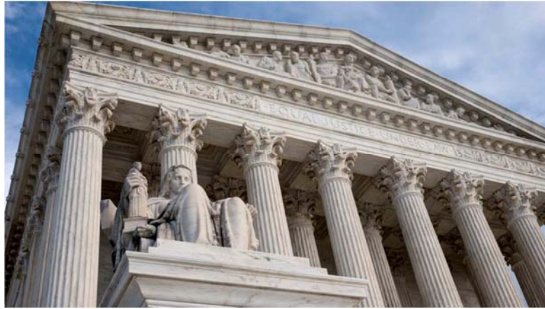
Figure 2. Is an example showing Roman columns used as decorative components, in addition to their main function as structural elements. Image is of the "Building of the US Supreme Court in Washington", Reference: [5].
