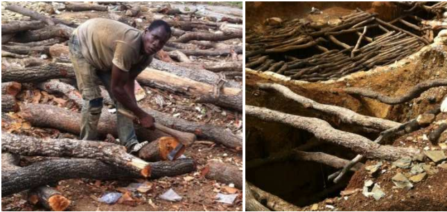
Figure 7. Trees cut from the savannah used to stabilize the walls of wells.
