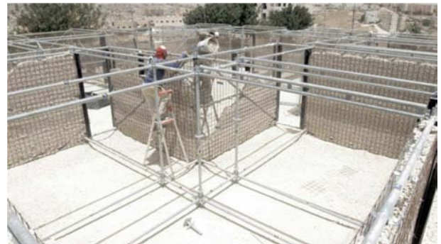
Figure 6. School for refugee children in Jordan, built with scaffolds and sand [1].
