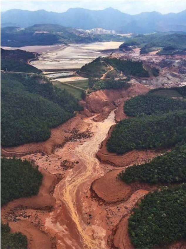
Figure 3. Fundão dam former site immediately after failure [2].
