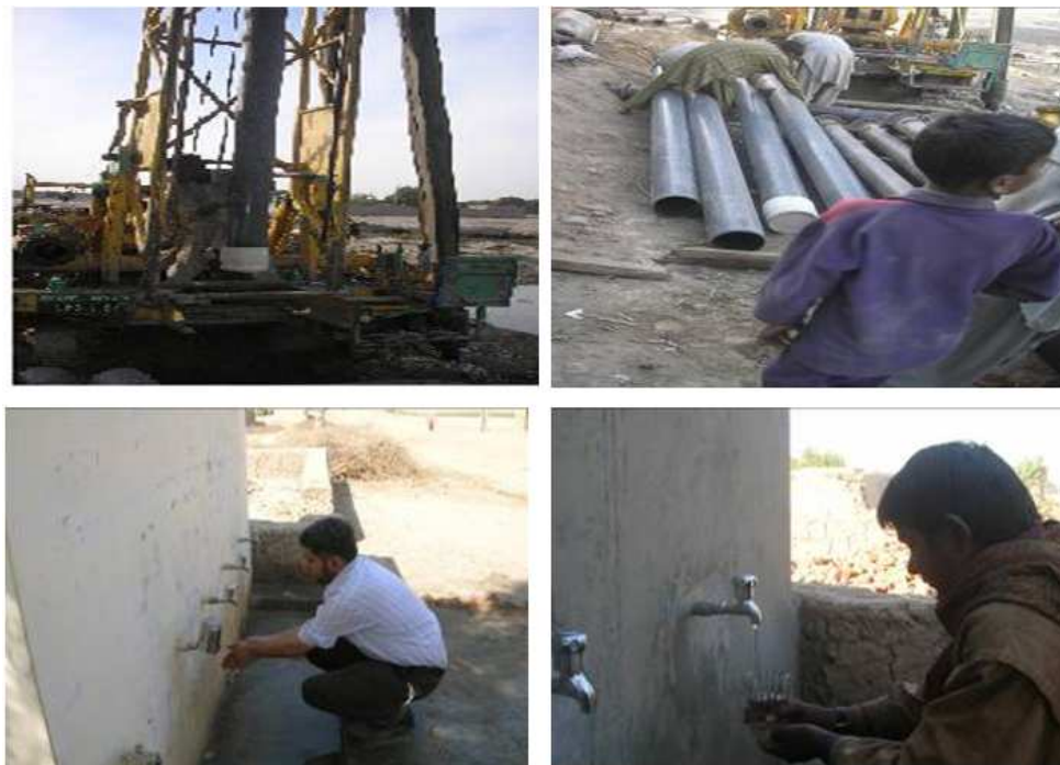
Figure 10. Deep bore hole upto the depth of 387 feet, which 10 ppb arsenic contamination which is within the WHO drinking water standard limits
