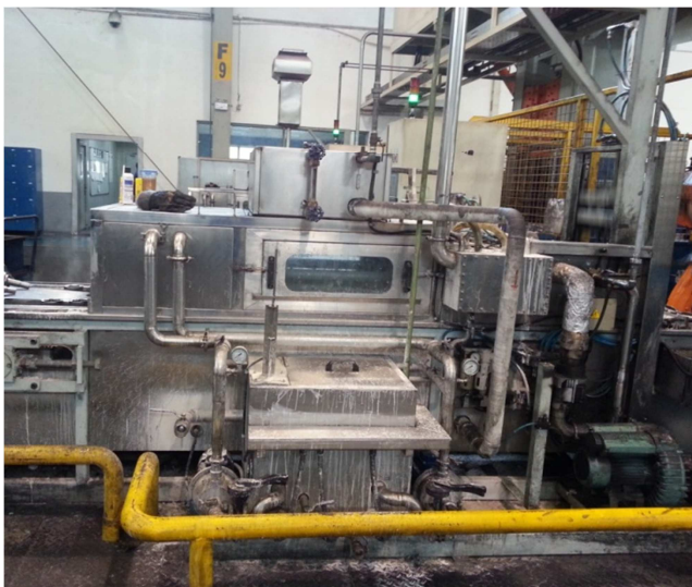
Figure 2. Saponification production line.
