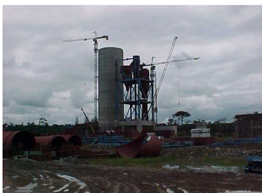
Fig 2. A cement plant (pre-heater plant) under construction in Nigeria.
