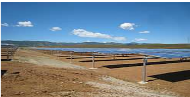
Fig. 4. Horizontal Single Axis Tracker in California.
