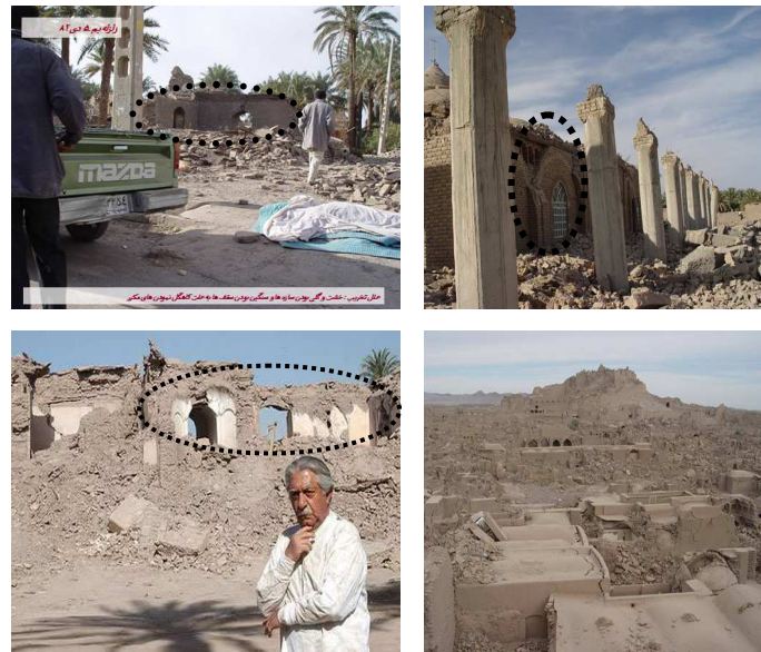
Figure (9). The remaining components are the result of a lack of concentration of stress and the arched nature of openings (Source: [4])
