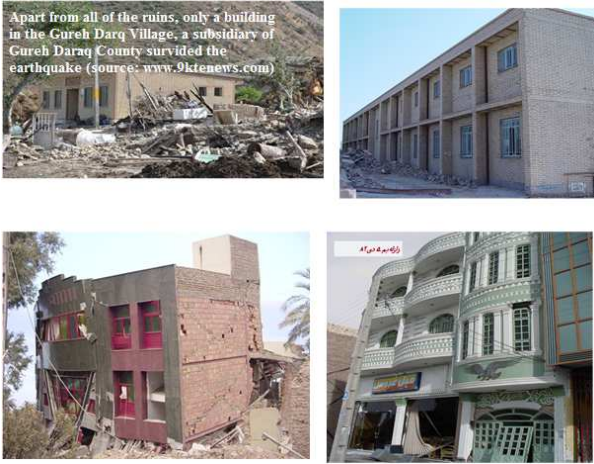
Figure (11). According to expert opinions, these buildings survived the earthquake due to the application of criteria for the design and construction of openings (source: [4])
