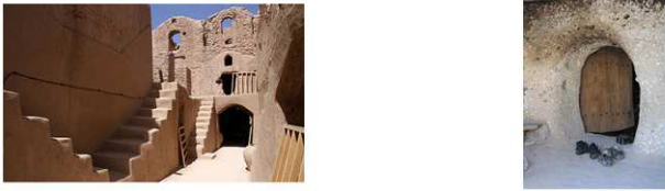
Figure (3). a) The fully arched gateways in the Meymand Village of Shahr-e Babak County, b) A gateway with vertical piers and an arched ceiling in the Sassanid fortress in Saryazd (source: www.goftarga.ir)
