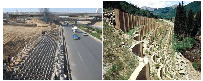
Figure 9. Examples of compound views (Right) the use of curved concrete walls (from: khakemosalah.ir ) (Left) the use of concrete cylindrical parts (from: parks.mashhad.ir )
