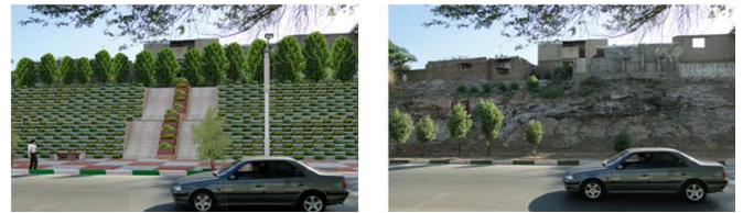
Figure 2. The role of reinforced soil in landscaping. (A) simple soil body – (B) modified body with reinforced soil (from: www.Ahvaz.ir)
