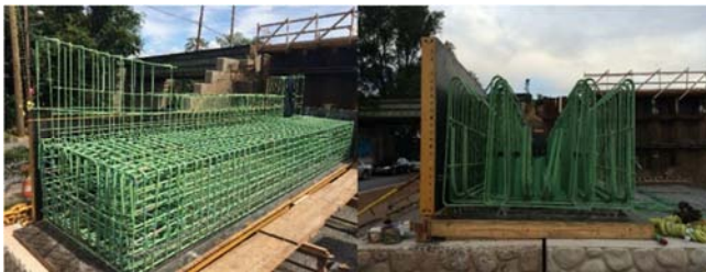
Figure 11. Tied on soffit rebar.
