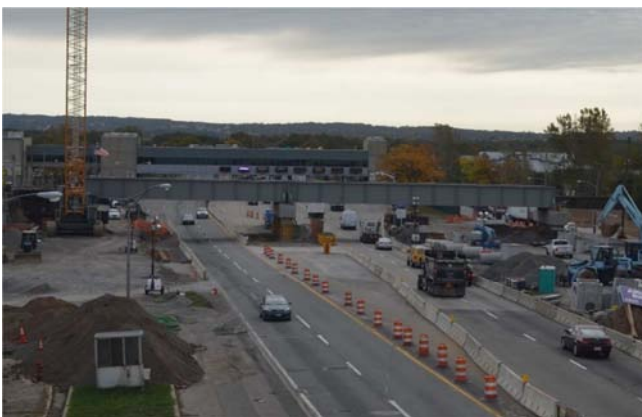
Figure 1. New Travis Spur Rail Bridge after the replacement weekend.
