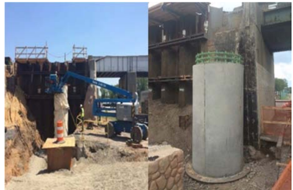
Figure 8. Wrapped forms for concrete thermal control (left) and completed pier (right).
