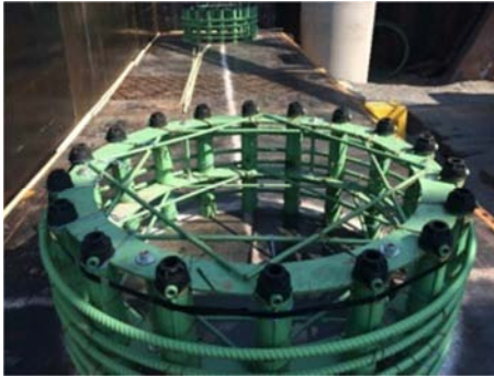
Figure 10. Rebar hoops placed around the couplers.
