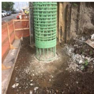
Figure 6. Rebar on top of the shaft.
