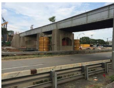
Figure 7. Formwork set around the rebar cage.
