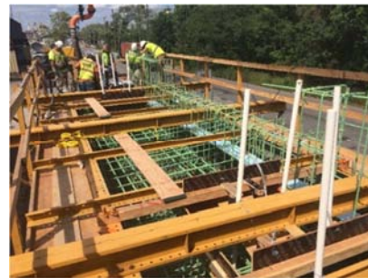
Figure 13. Casting of the cap beam using a pump truck.
