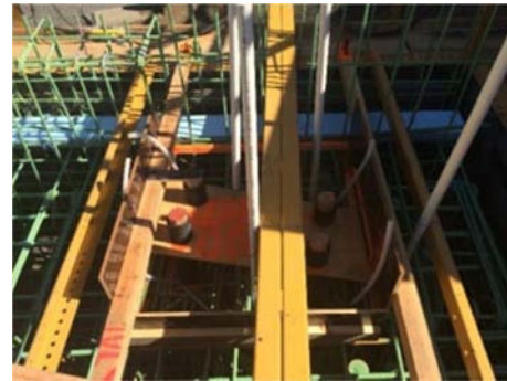
Figure 12. Pedestal forms with anchor bolt sleeves.
