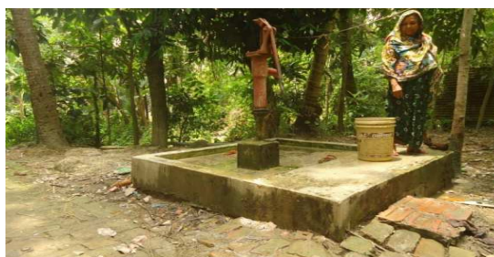
Figure 11. Raised Water Pump for drinking water security during disaster.
