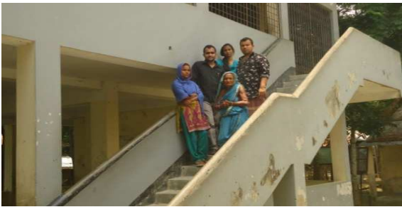
Figure 12. Cyclone Shelter in Angaria Union.
