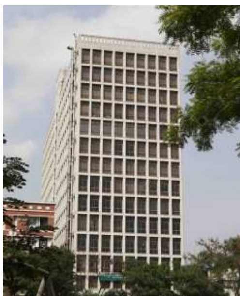
Figure 2. ASA Head Office.
