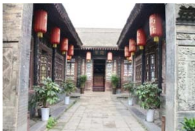
Figure 3. Bei Yuan Men No. 144 Gao courtyard [11].
