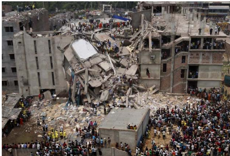
Figure 10. Savar Rana Plaza building collapse (Source: New Age Online , 2013).
