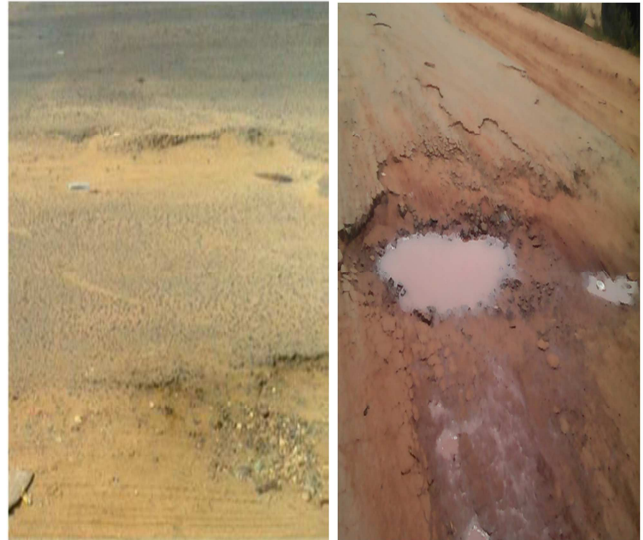
Figure 1. Deteriorated Parts of the Road.
