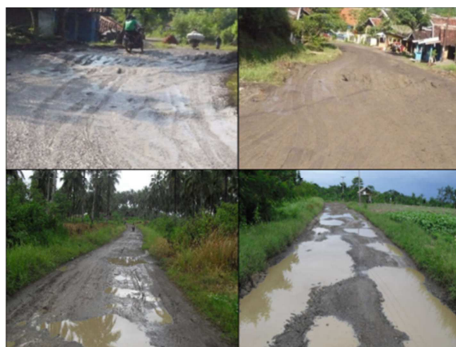
Figure 2. The condition of existing roads in the southern part of West Java before hardening with CTB.
