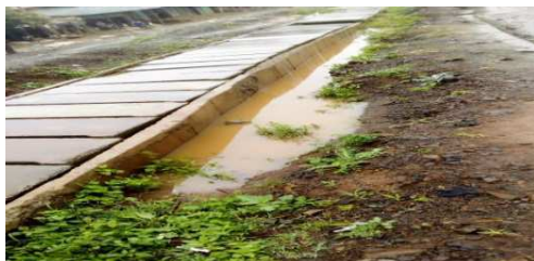
Figure 8. Ponding sides of U-ditch at Gessa Town (photo: by Mengistu Bayu, 19 th May, 2021).
