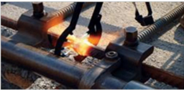
Fig. 5. Head to head forging welding.
