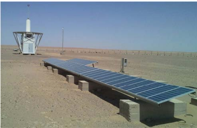
Figure 9. Solar energy system to operate radio navigation station for aircraft in Dongola International Airport.
