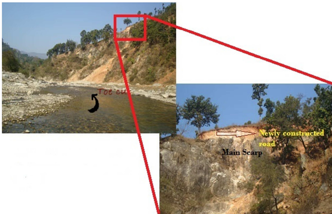
Figure 5. Unstable slope of the Robang Formation; Toe cut and newly constructed road damaged (right).
