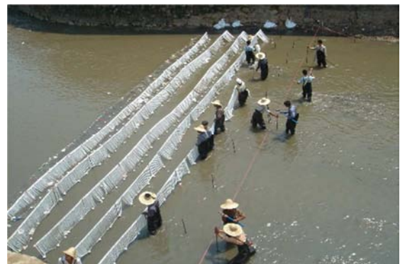
Figure 8. Installation of braided shade soft filler in river.
