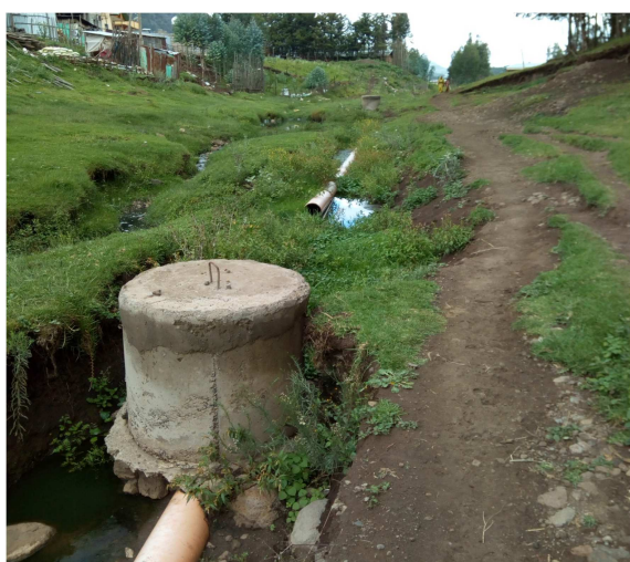
Figure 5. Broken sewerage pipeline causes land slide.
