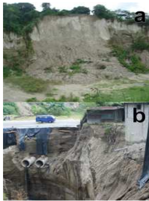
Figure 1. Mass wasting problems in Tierra Blanca Joven (TBJ). a) corresponds to las Cañas River where mass movements, erosion and collapse occur all the year. b) Is a 2005 photo of a stream in Ilopango, the landfill and pipelines of the road failed during heavy rains of hurricane Stan.
