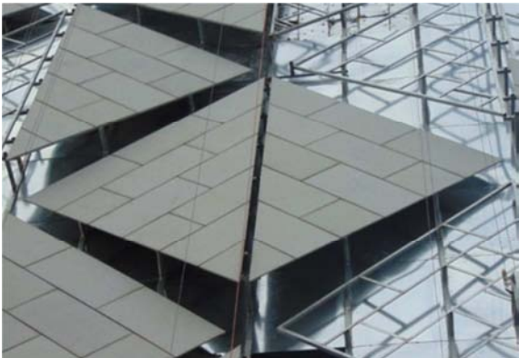
Figure 8. Picture of installing process of composite stone simply supported on four sides.
