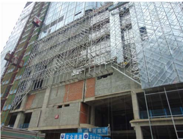
Figure 12. Picture of stone sub-keel triangle frame installation.
