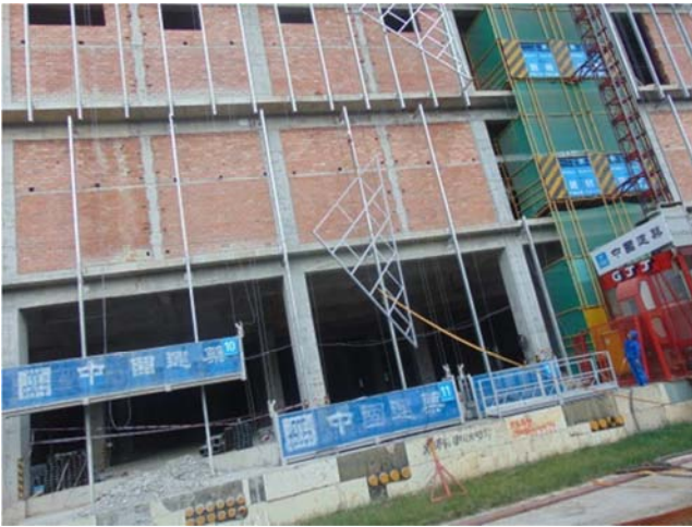
Figure 11. Overall lifting of triangle frame.
