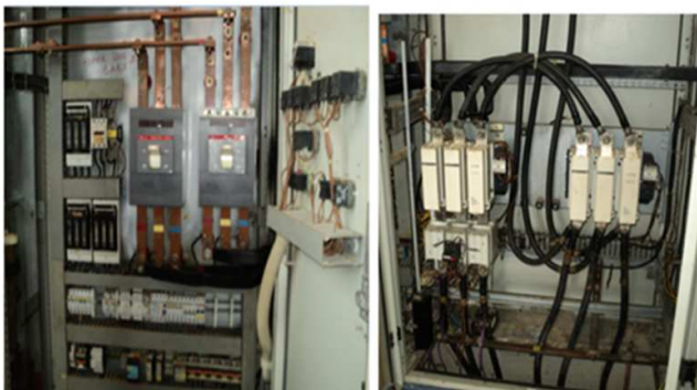
Figure 2. Charred Electrical Installation.
