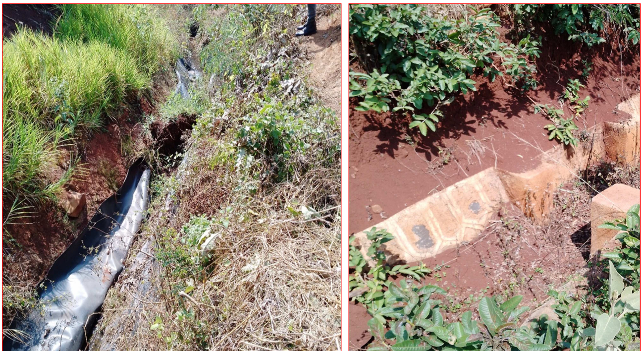
Figure 2. Canal filled with sediment at Seka-Chekorsa district on Gibe-Kechema Scheme.
