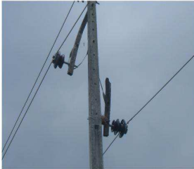
FIG 3. 11Kv line with a Slanting cross arm.
