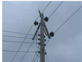
Fig 4. 11kV Line with a cross arm.
