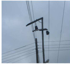
Fig 2. Wooden Pole with a Broken Wooden Cross-Arm.
