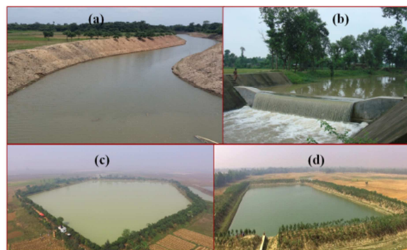
Figure 5. (a) a re-excavated canal, (b) a cross dam (check dam) in the re-excavated canal, (c) a re-excavated pond and (d) re-excavated portion of a natural beel..
