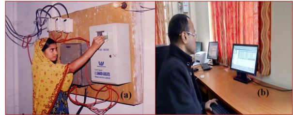
Figure 10. (a) a lady farmer is inserting her prepaid card into the prepaid meter of the irrigation equipment and (b) The total system is being monitored from the head quarter of BMDA using internet net work.
