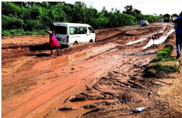
Figure 3. Failed portion of Itobe-Ajaokuta Expressway.
