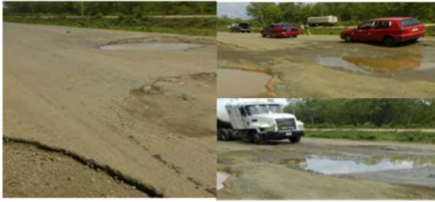
Figure 2. Failed Portion of Itobe-Ajaokuta Expressway.
