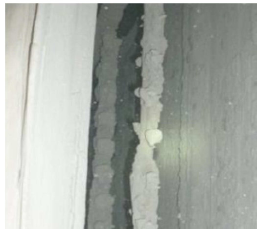
Figure 10. Dust Accumulates in Electric Precipitator.
