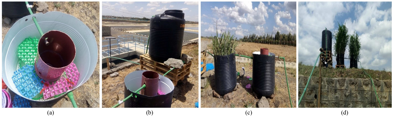
Figure 2. (a) Tank with prefabricated tubular blocks for plant support and filter column (b) Connected tanks before introduction of plants and filter (c) Typha latifolia planted in Tank 1 (d) Complete FTW system.
