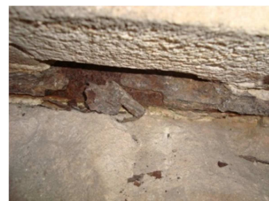
Figure 4. Corrosion products resulted in stone fall down.
