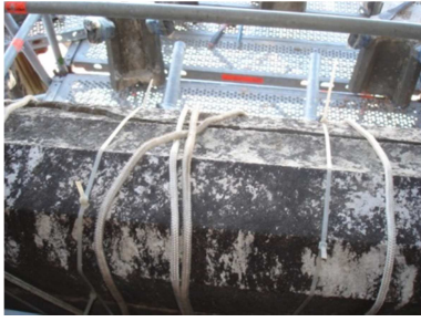
Figure 5. Detached parts kept temporary in position by ropes.
