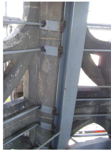
Figure 10. The columns of the steel structure and its connections with the spire.
