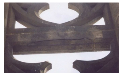
Figure 3. Wide cracks due to corrosion products.
