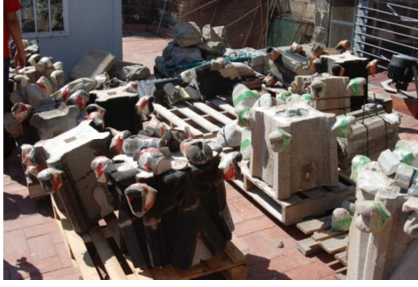
Figure 6. Storing the dismantled parts on the cathedral roof.
