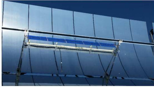
Figure 12. MH Solar CSPV system installed at the UL Lafayette START Center.
